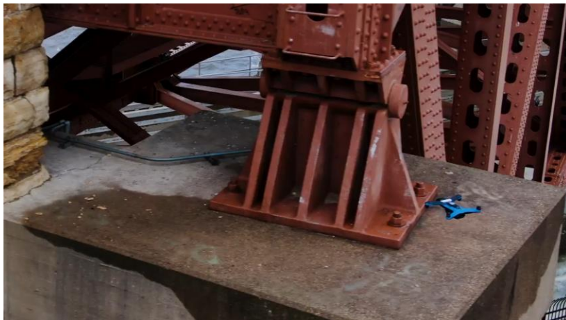
SKYDIO: Bridge inspection
